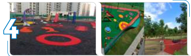
Colored granules mixed with PU binder/ application
