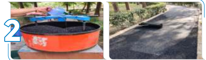
Mixing SBR Granules/ Laying of base layer 9 to 44mm
